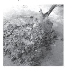
If the mortar is too dry it won't spread or stick to the blocks properly. If it is too wet, the water will separate from the sand and the mortar will run off the blocks.
