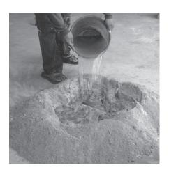
5. Lift the dry mix into the water — a little bit at a time until all the water is used up
