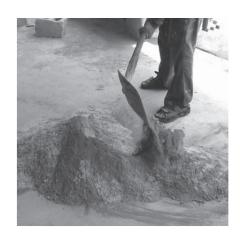
3. Make a heap of the mix and make a hole in the middle
