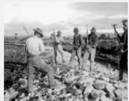
Road construction c. 1910. ALEXANDER TURNBULL LIBRARY, REF. G-10600-1/1.
