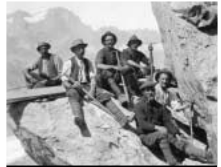
Carrying timber up the Tasman Glacier to build the Haast Hut, 1915 – 16.
