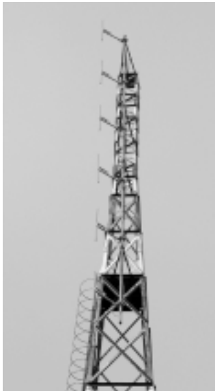
Fig 9. Dipole Antenna System
